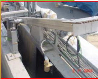
NR- Manual Screens Georgian Downs Racetrack, Barrie, ON Design Flow: 82.6 m 3 per day
