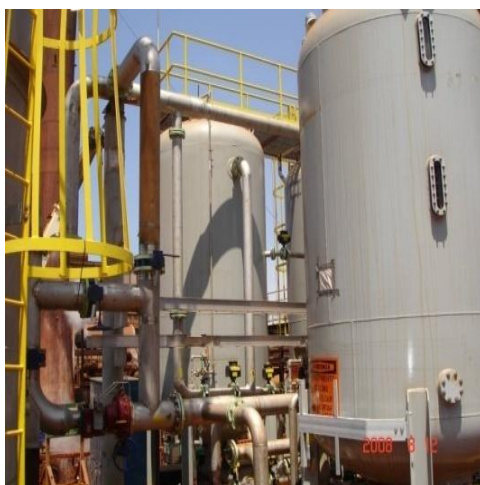
Ion-Exchange Demineralization Moa Nickel, Cuba Design Flow: 6720m 3 per day
