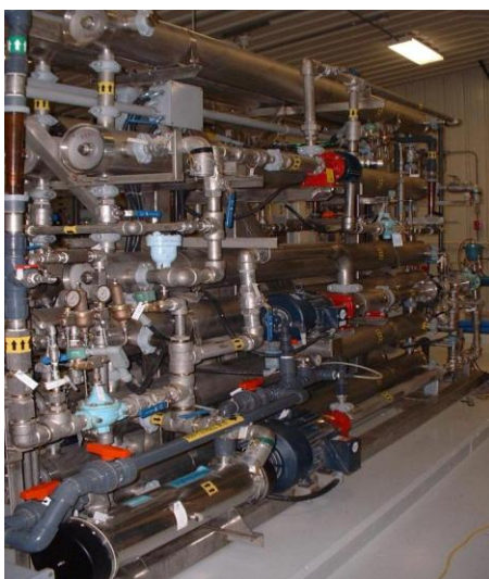
Nanofiltration System Pelican Falls, Ontario, Canada Design Flow: 280 m 3 /day
