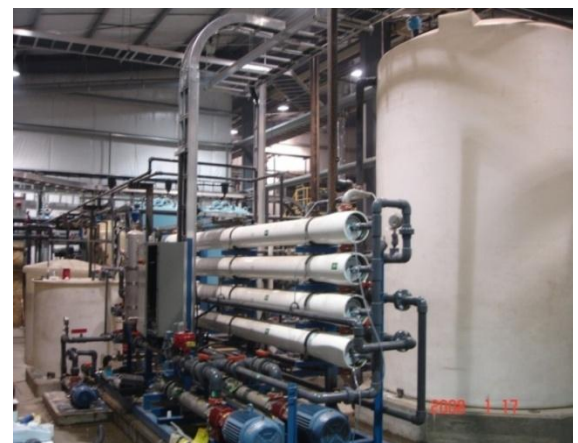
RO System Tolko Industries, Alberta Design Flow: 380m 3 /day
